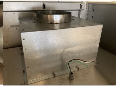
24. Once the insert is secured, connect the electrical wiring and duct piping through the hood body front opening.
