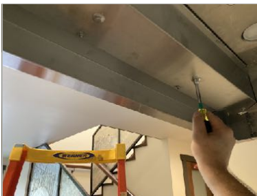
28. Re-secure the front panel using the supplied M5x15 screw hardware while pressing the bottom of the panel rearward.
