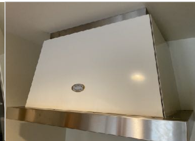
27. Re-install the hood body front panel by hooking the top lip centered over the upper panel support bracket.
