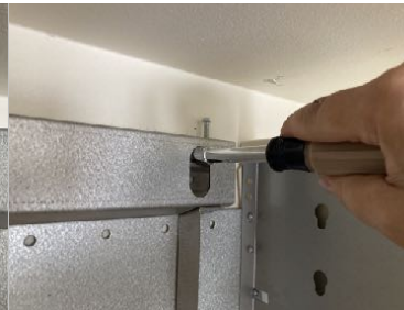
17. Hand tighten the M6x30 screws lightly to flatten the hood body to the wall but to still allow movement.
