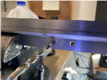
14. The hood support bracket may not align stock mounting holes to wall studs when centered, drill new mounting holes in the bracket to target the center of the wall studs as needed.
