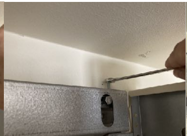
18. Level the hood body by tightening or loosening the (2) left or right M5x40 screws.
