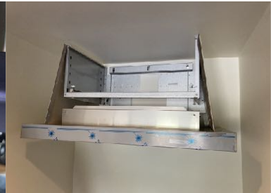
15. Hang hood body centered on support bracket and level unit using the (2) M5x40 leveling screws.
