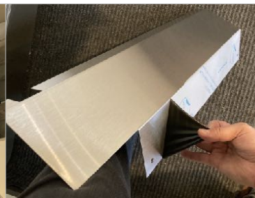
29. Peel the protective laser-film from all the finishing trim panels.
