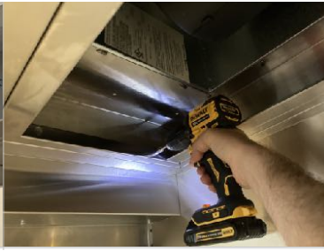
23. Install Motor/Blower Insert flush to the underside of the hood mounting flange using SS self-tapping screws.
