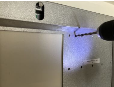
20. Screw the rear body to wall into studs where possible near the top and bottom of the rear panel. Drill new holes through panel as needed to align to studs.
