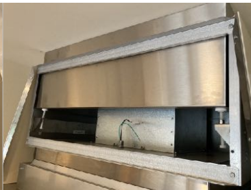
26. Reinstall the front panel support bracket(s). Make sure the bracket fixes the body side panels as wide as possible at the top.
