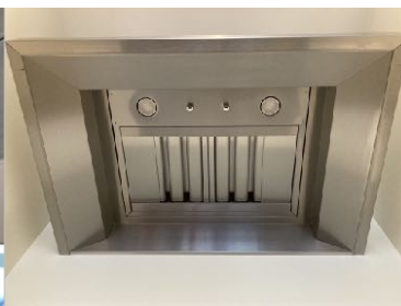
32. Install Motor/Blower Insert filter baffles and spacers to center the filters.
