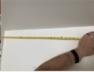
11. Measure and mark the mounted hood body centerline at the support bracket mounting location.
