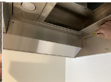
30. Install the left and right side finishing trim panels first. Secure panels with one of the provided screws only at the rear of each panel.
