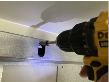
19. Once level, secure the hood to the wall by fully tightening the M6x30 screws. This pulls the rear panel to the wall.
