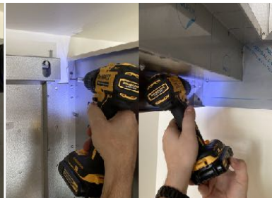
21. It is imperative to secure the upper and lower hood body to corners to the wall with the appropriate screws. Use both mounting holes provided.
