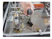
7. The 120v solenoid will make a slight buzzing sound while under electrical load. If it is silent when all other components are under correct operation and electrified, remove and replace by unscrewing it from the main valve body by removing the 13mm nut & washer. It will slide forward off the magnet shaft. After it is off the end of the shaft, turn it upside-down and remove the Philips screw. Unplug the connector and replace the solenoid. Install in reverse order.
