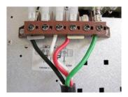
1. Check the terminal block connections. Make sure all terminal screws and jumper bars are in place and tightened.
